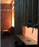
Figure 5 : Interior kids bedroom with both timber slab and timber partition wall
