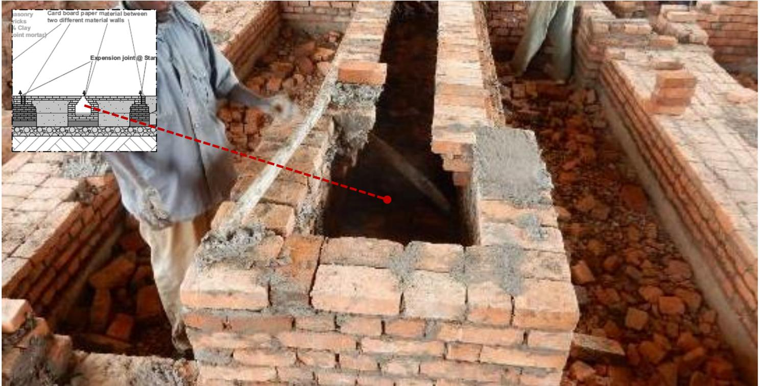
Smoke tunnels are built simultaneously with external walls, using semi-refractory bricks. 42,000 semi refractory bricks are required for the entire kiln (10days)
