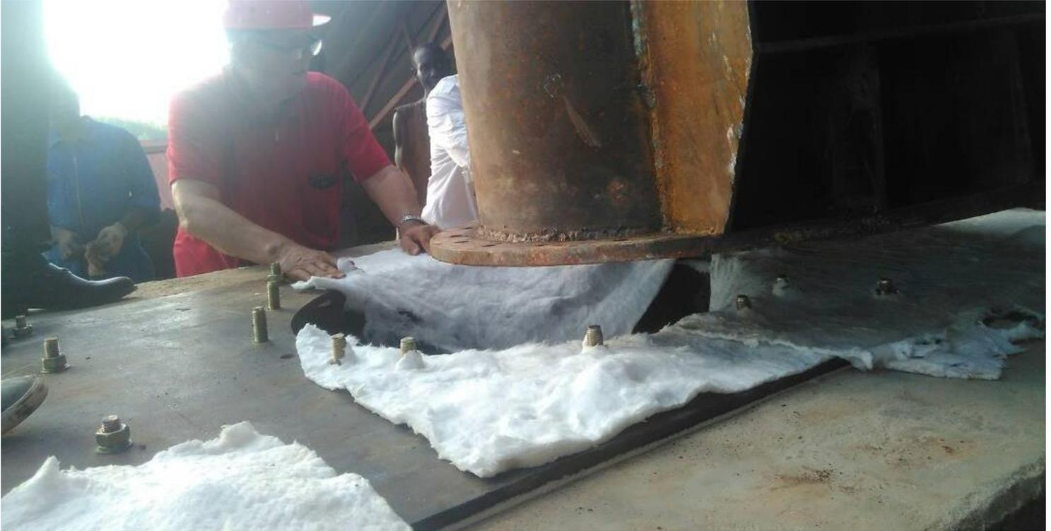
A fire proof fibre matt is placed on top of fire control box to seal gaps between the box and the chimney.
