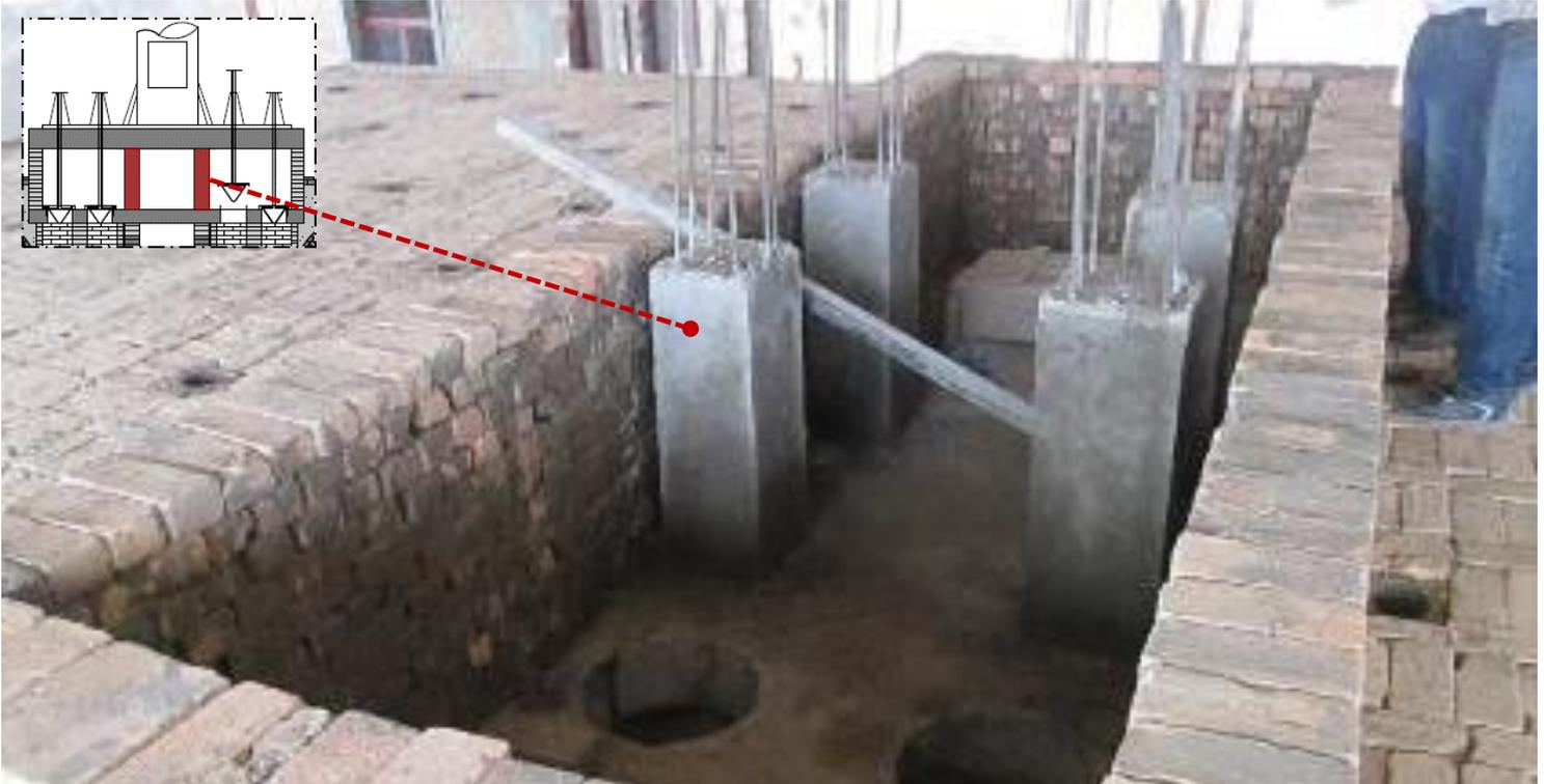
The fire control box has 4 R.C columns in the middle for supporting the chimney. Columns cast within (3days).
