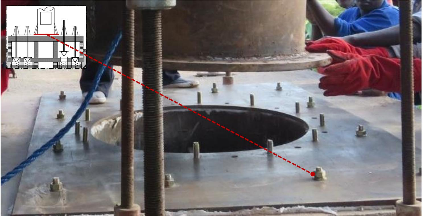
The chimney is fixed to the kiln by means of bolts and steel plates concreted and anchored to the fire box R.C roof and columns.
