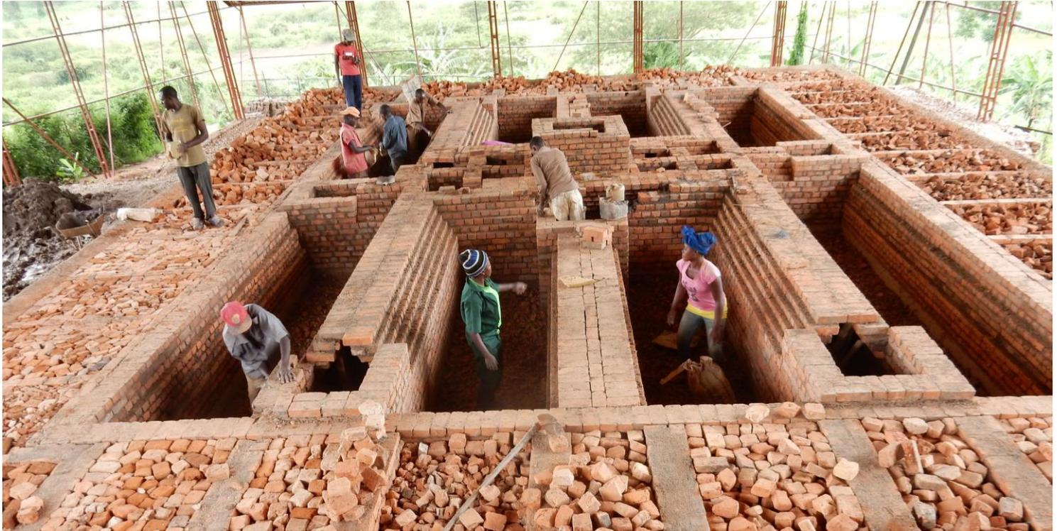
Kiln construction at floor level with the smoke tunnels in place
