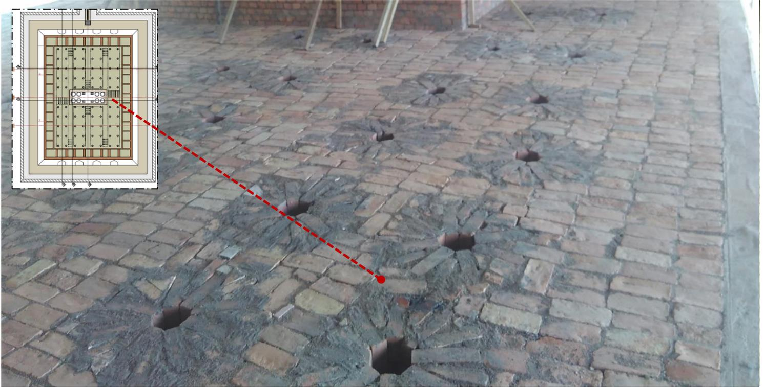
The kiln top is built with 2-layers of dry-stacked bricks following the pattern illustrated above. (3days).
