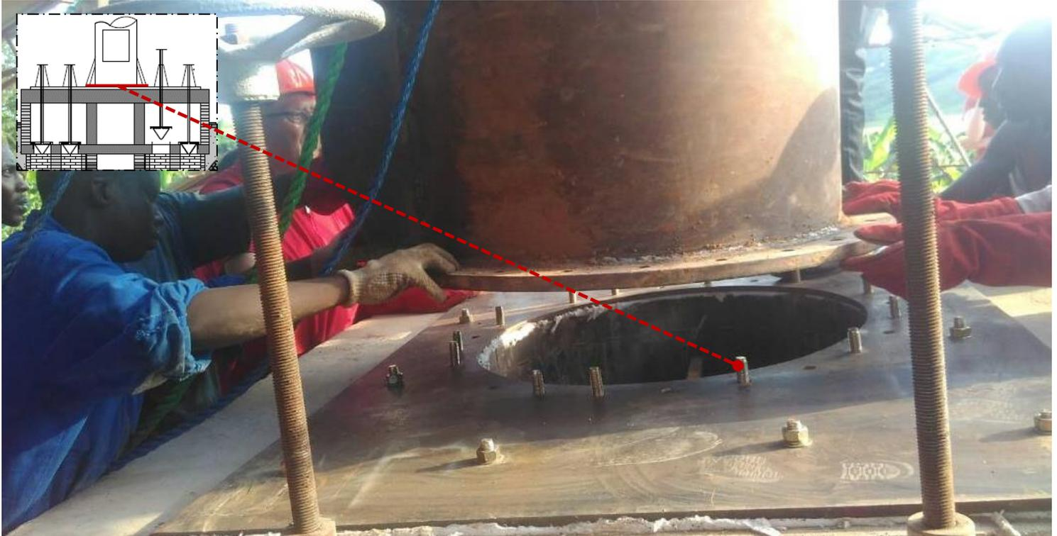
The chimney is fixed to the kiln by means of anchor bolts concreted on top of the fire control box.
