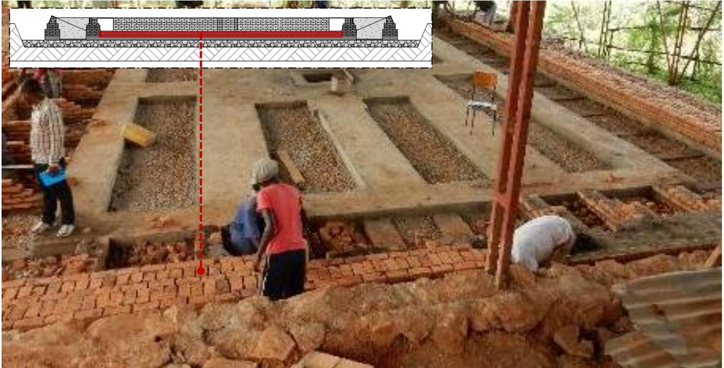
Building external walls to ring beam (10days). Joints should not exceed 5mm. 83,600 bricks are required for the entire external walls.
