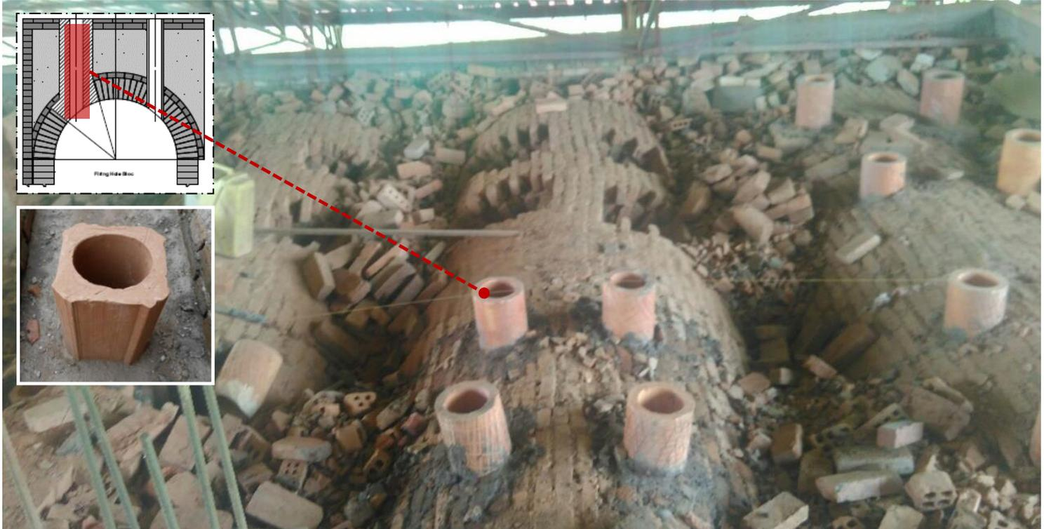
Fuel feeding bricks are inserted in place, creating the holes for feeding the firing fuel. 160 pieces of such bricks are required.
