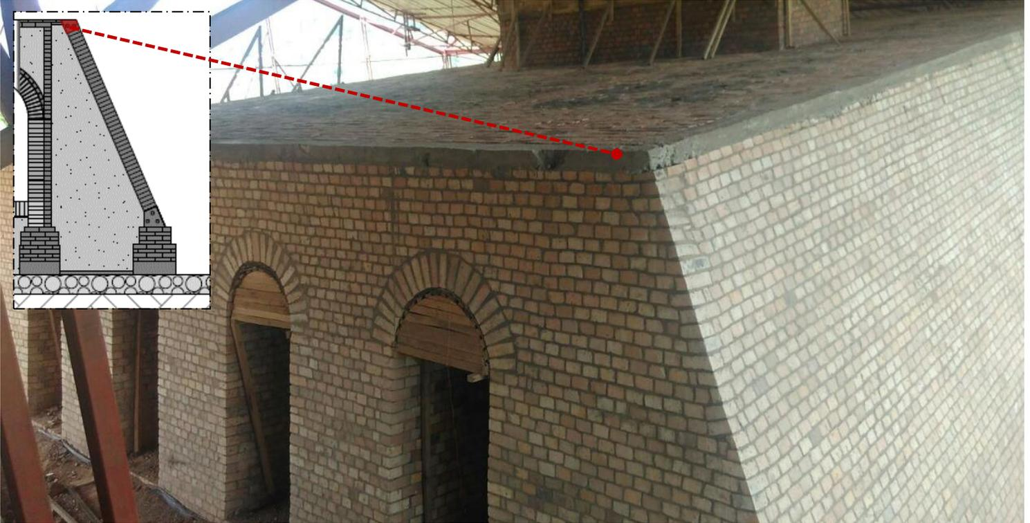
A R.C Top Tie is cast around the top of the kiln to hold it together. (2days)
