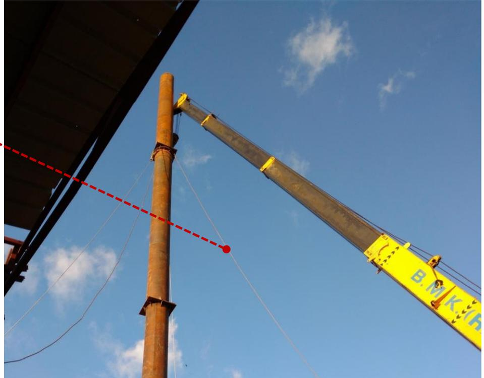
The chimney is braced with 4, 16mm (Total 120m) steel cables anchored to concrete columns. (1 day).
