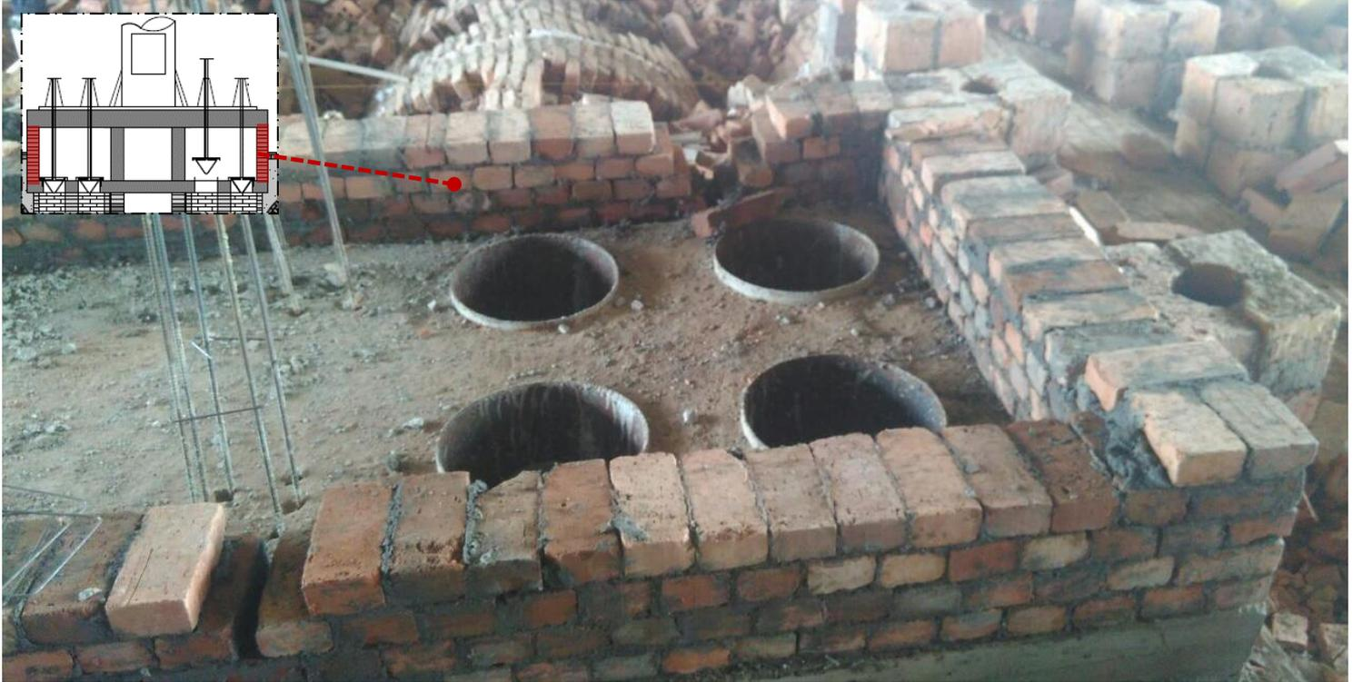
The fire control box with the steel reinforcement for the columns, and the fire control holes in place. Building walls to kiln top (5days).
