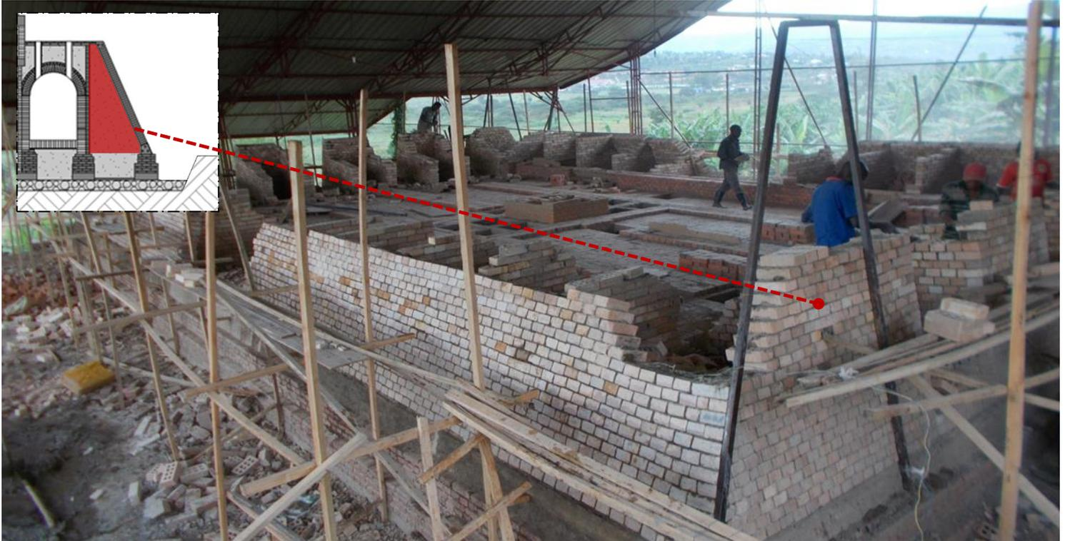
All the gaps between walls are filled with well compacted broken bricks as wall construction progresses. (10days).
