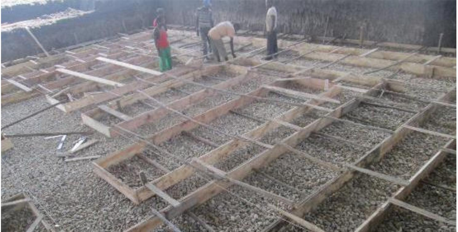
Formwork to support concrete pads for kiln foundation is erected accurately, set as per specifications. (2days).
