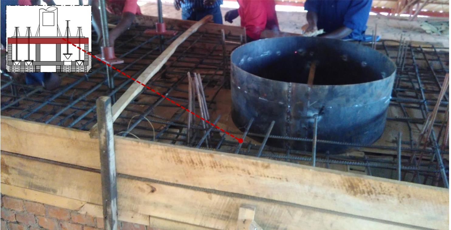
The R.C roof slab where the chimney rests.
