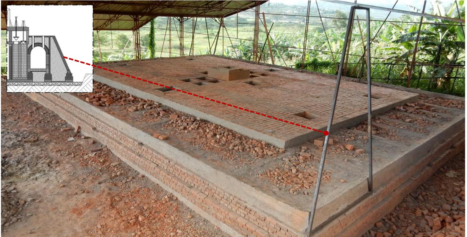
A metal or timber frame is made to guide in building the kiln slanting wall.
