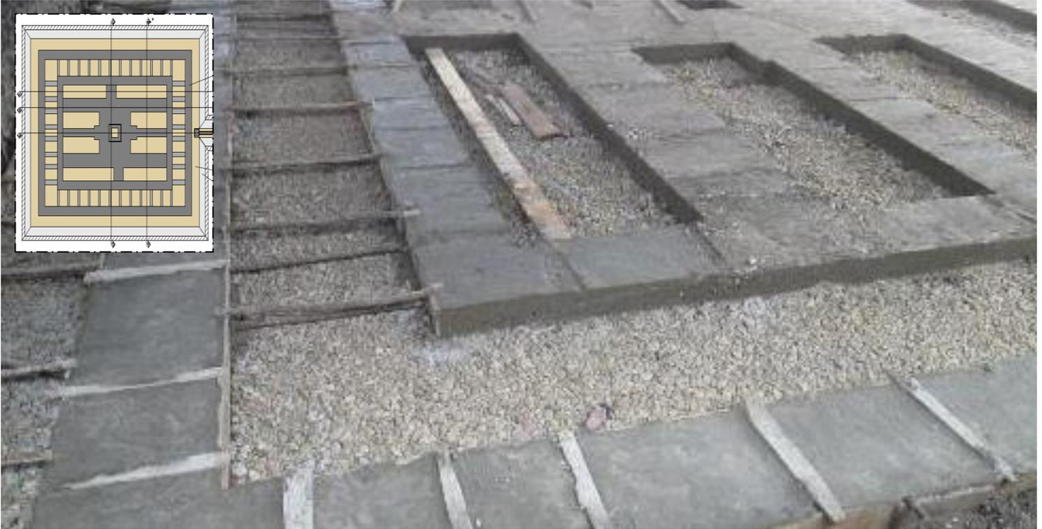
18m<sup>3</sup> concrete (1:2:4) is poured inside the formwork (2days).
