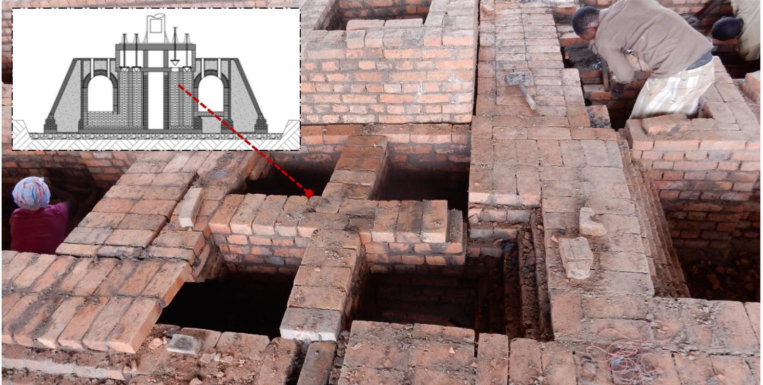
Joints between bricks should not exceed 5mm and are filled with clay/ kaolin/ chamotte mortar. (7days)
