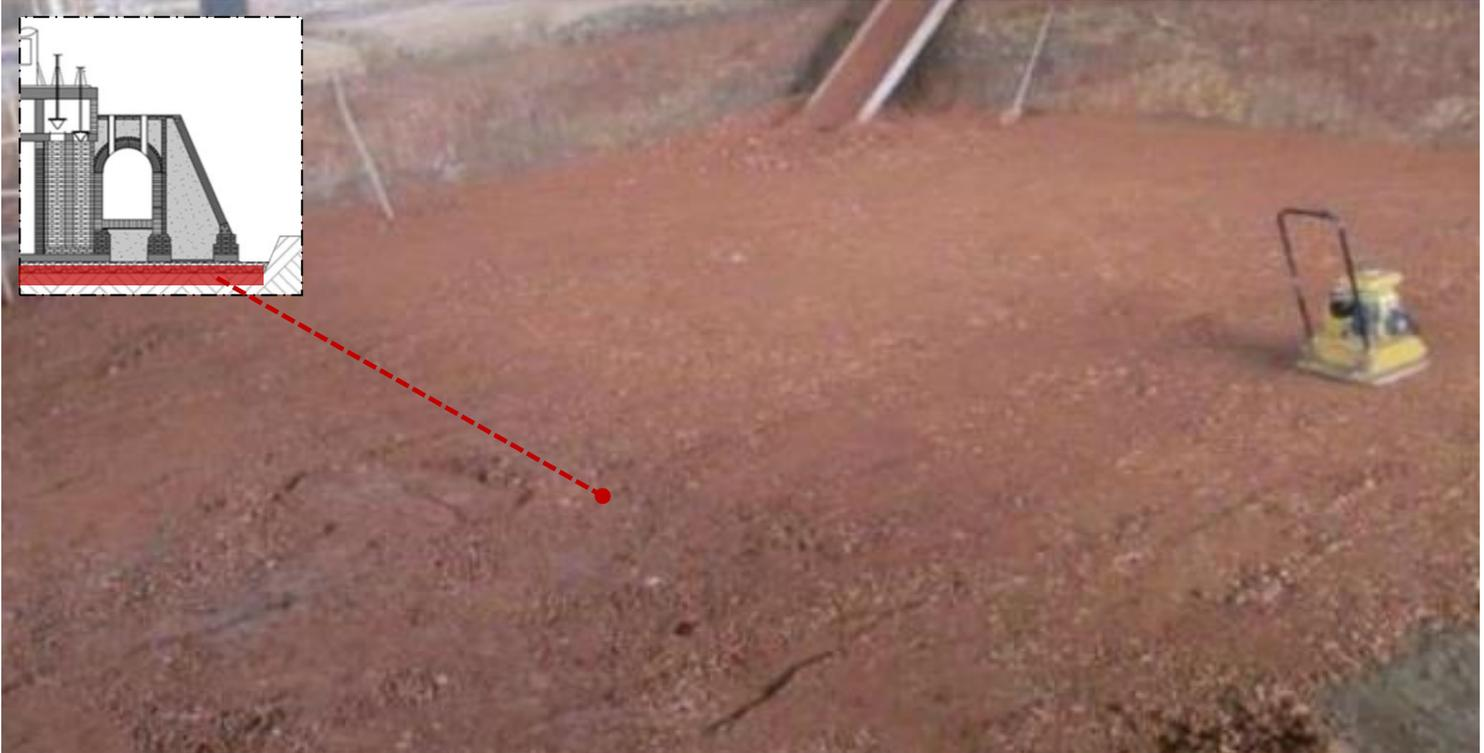
If the sub-soil at 1.04M depth is not stable enough, good soil (50M<sup>3</sup>) such as laterite must be brought and compacted to 2Kg/cm<sup>2</sup>, 200mm thick. (2days.)
