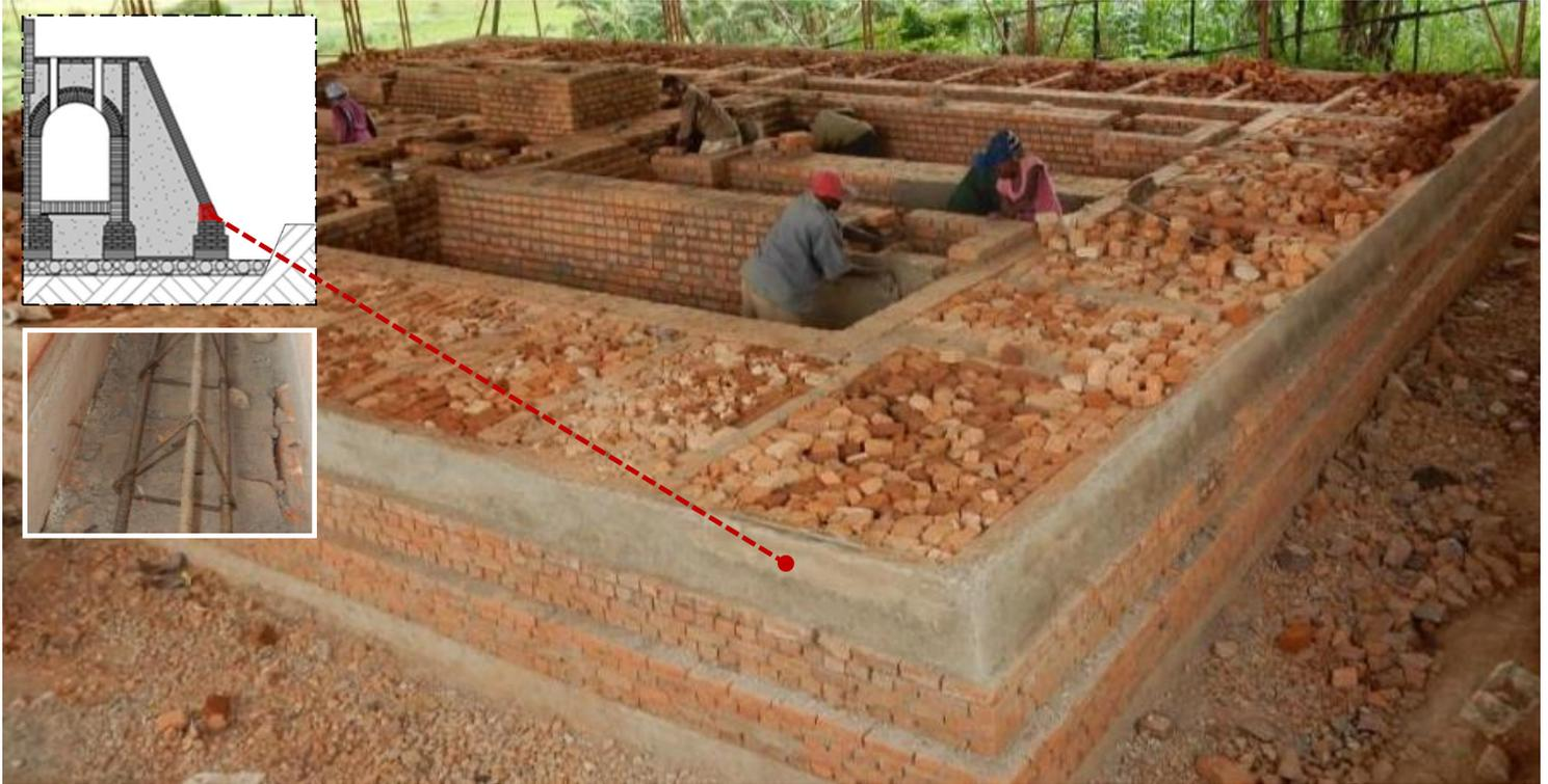
Casting the Ring Beam. The concrete ratio for ring beam is 1:2:4, The ring beam is reinforced with (3), 12mm steel bars tied with 6mm stirrups.
