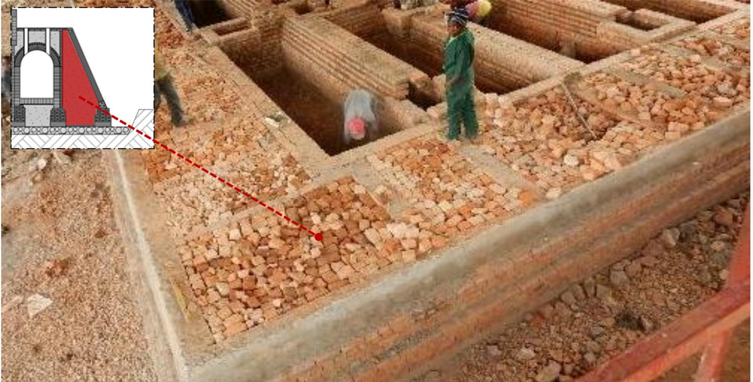
Approximately  $73\text{M}^3$  of broken bricks is required for backfilling the various sections of the kiln. (3days).
