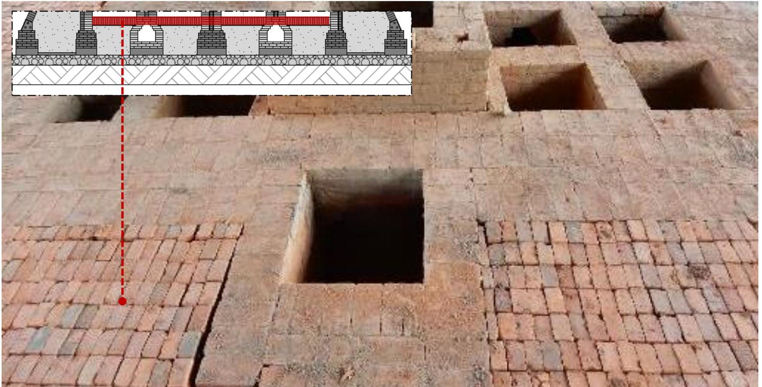
The kiln floor is built with semi-refractory bricks laid vertically (soldier course). (5days).
