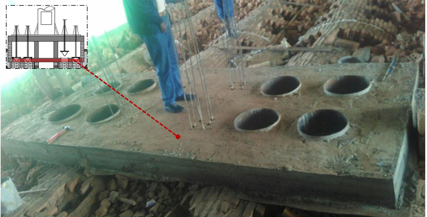
The fire control box is built in the middle of the kiln, where all the chambers and chimney are connected. Formwork and slab casting (5days).
