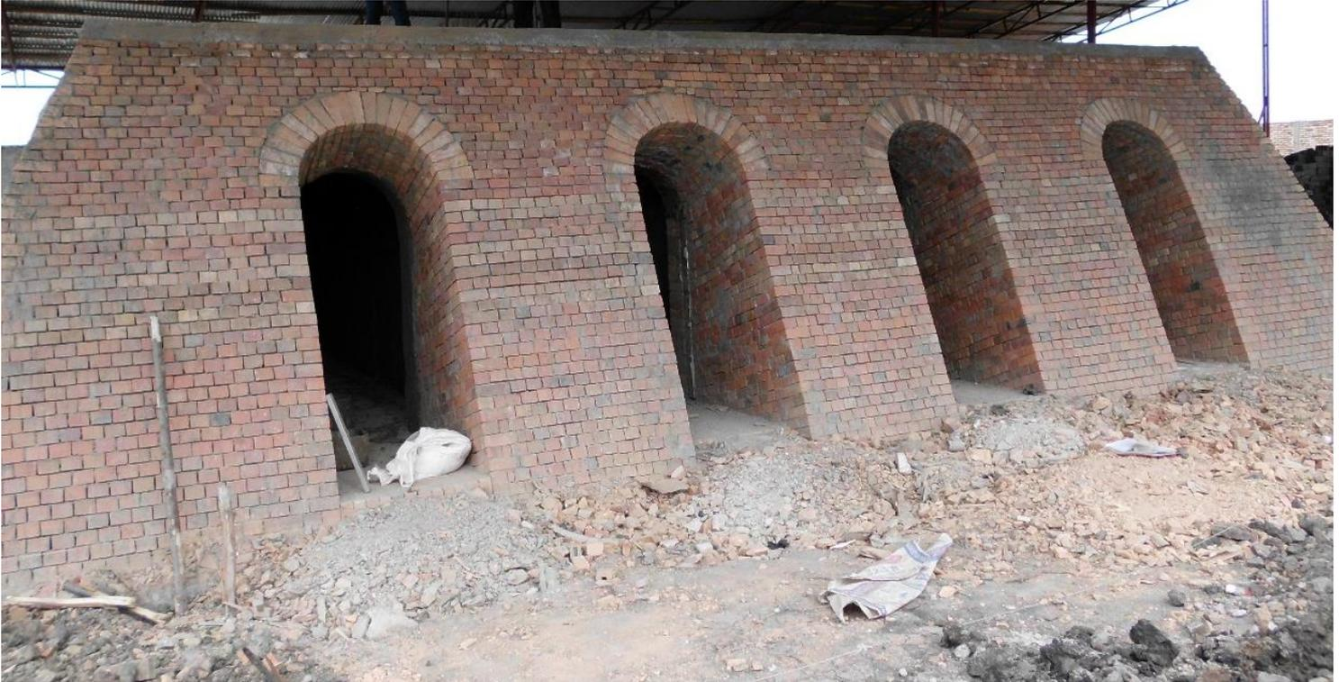
Brick laying of external walls are laid to the top of the kiln, tied together by a R.C tie beam.
