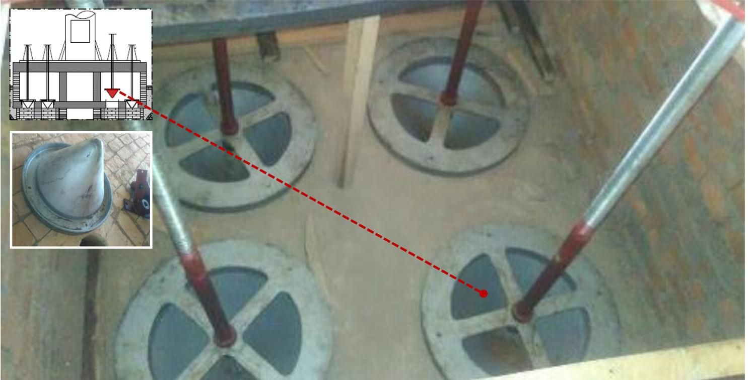
The fire control valves installed in place. (2days)
