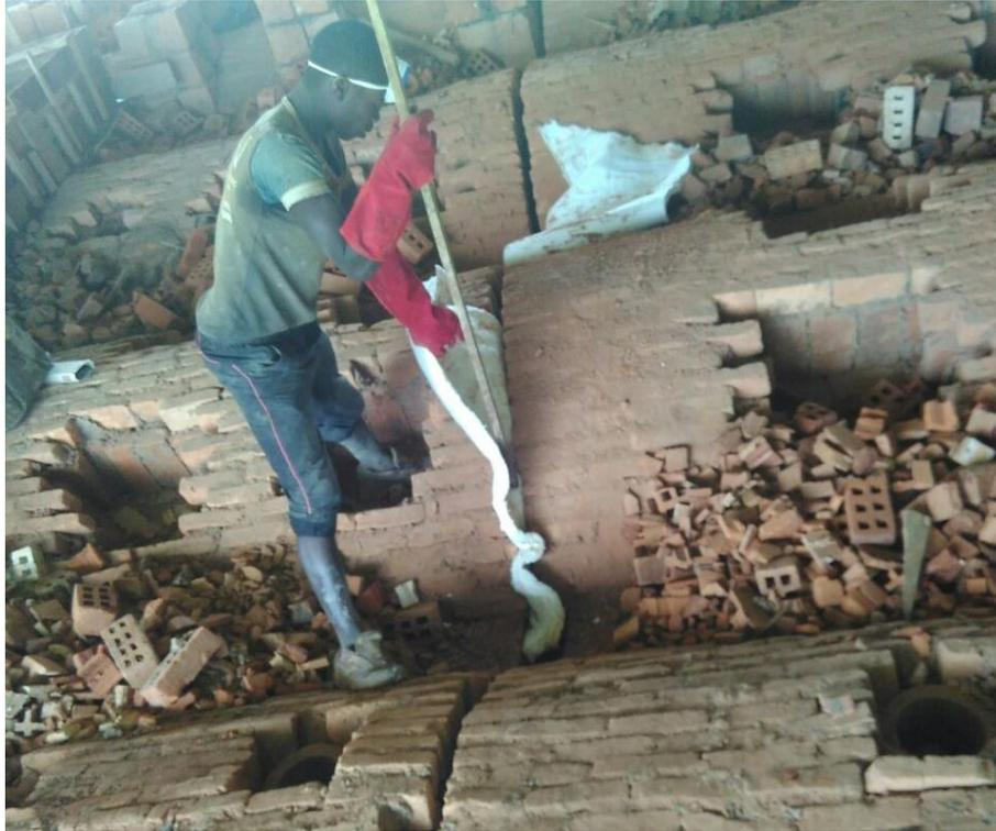
Expansion joints in the vaults are sealed with fire resistant material. There are 6 expansion joints, one in each vault.
