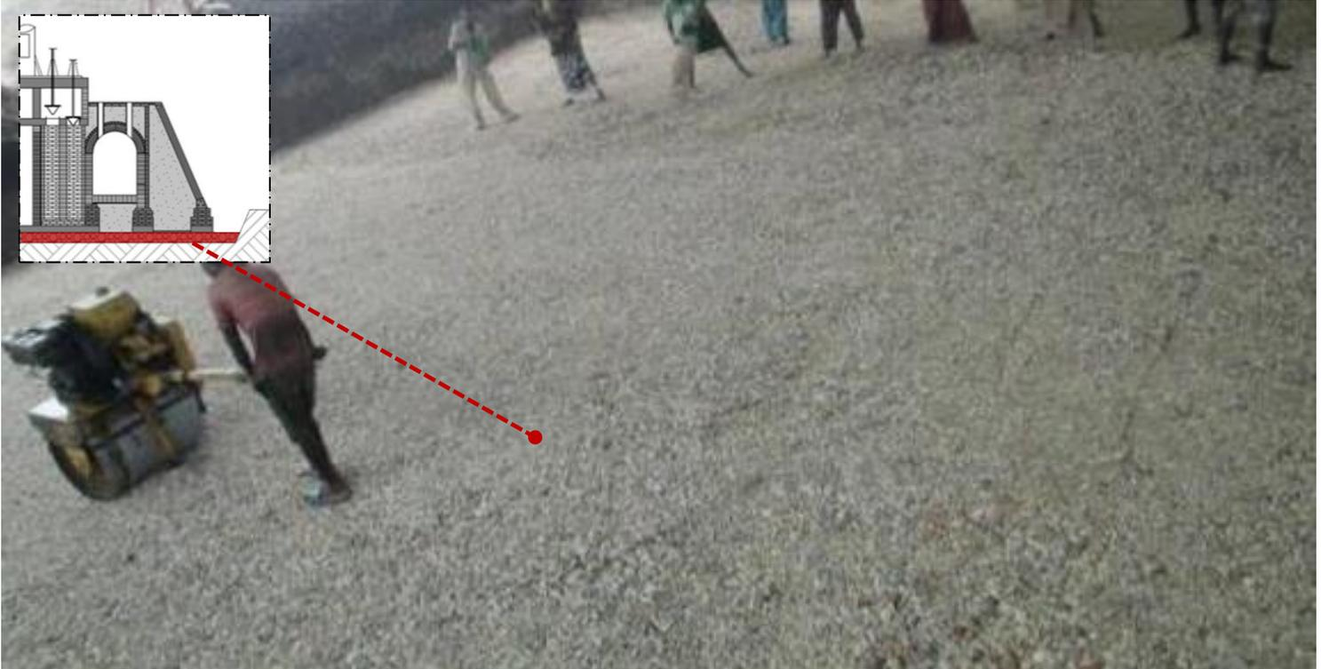
A 20-40cm thickness layer of gravel is compacted for drainage purpose. Approximately 112M<sup>3</sup> of Gravel 15-40mm thick is required. (2days).
