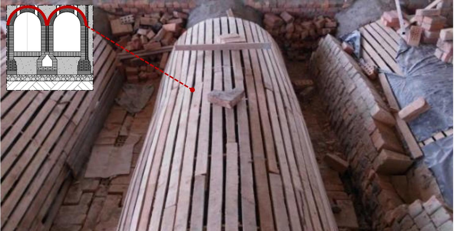
Kiln chambers are bridged with vaults. The vaults are supported with wooden formwork. (5days).
