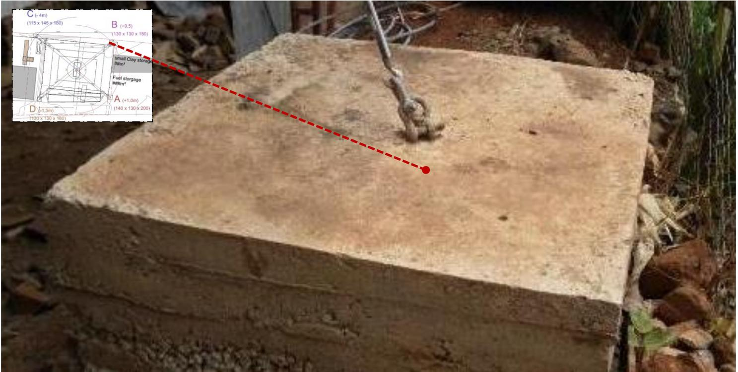
Four concrete columns are cast at specified corners for anchoring the chimney to the ground. (3days).
