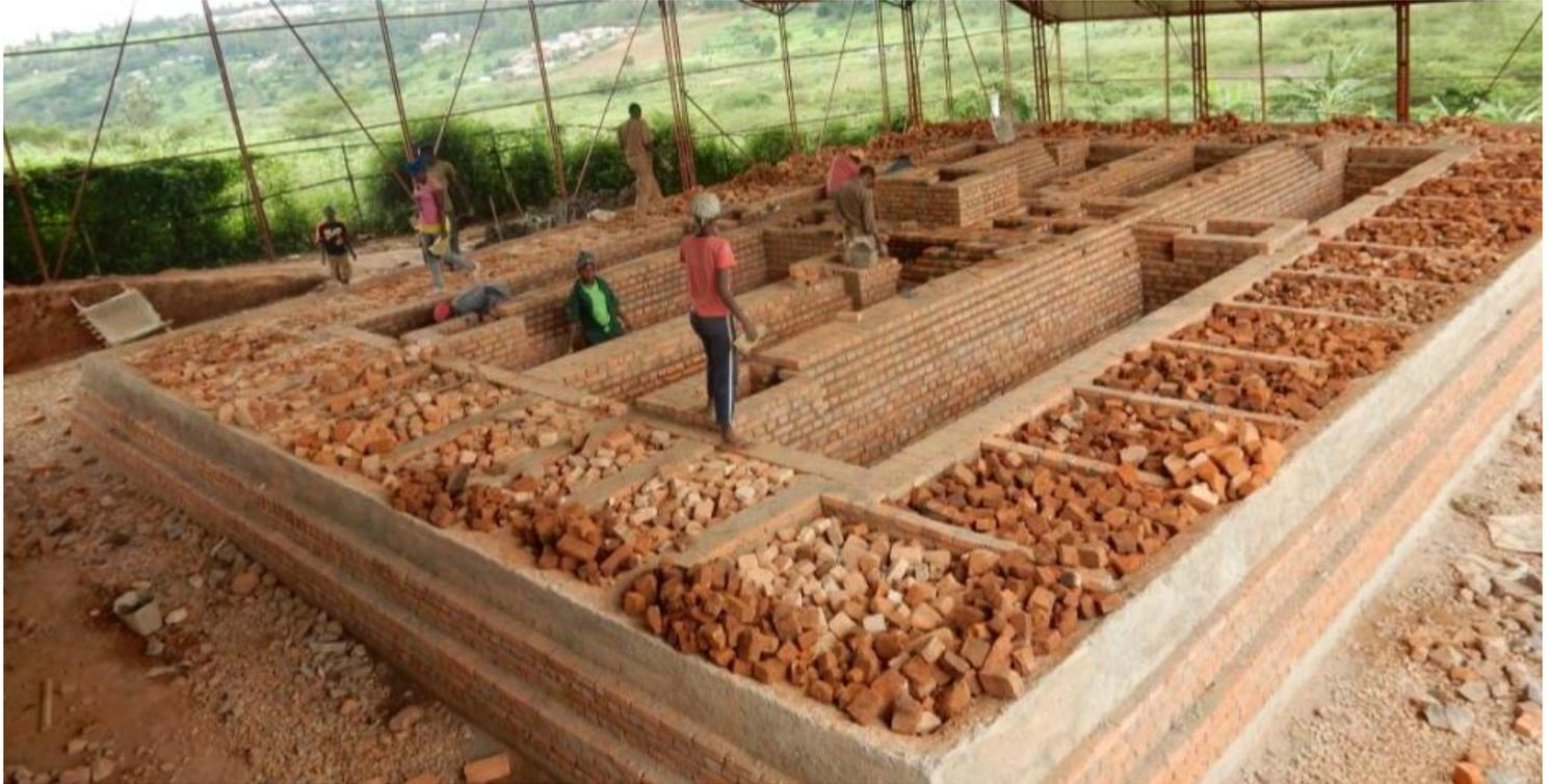
Backfilling with approved materials such as hard broken burnt bricks for insulation.
