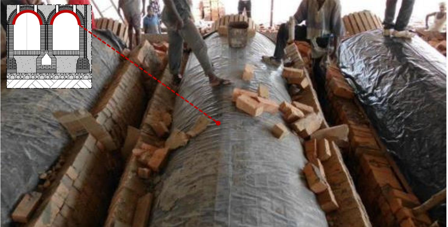
The vault wooden formwork is covered with polythene sheet to prevent leakage of the liquid mortar.
