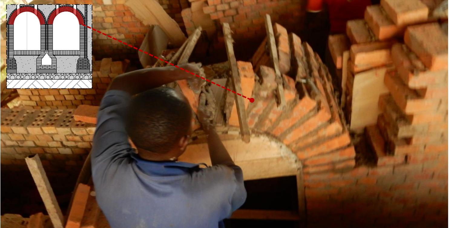
The vaults are built with special wedged refractory bricks with joints filled in clay/kaolin/chamotte mortar.(10days). 26,000 bricks are required.
