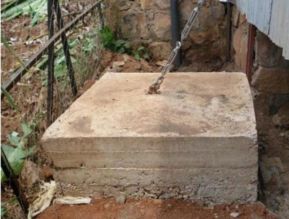
The chimney is anchored to the 4-concrete cubes. (1 day)
