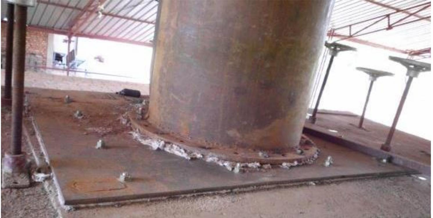
The chimney is bolted in the steel plate anchored to the concrete slab. (1 day)
